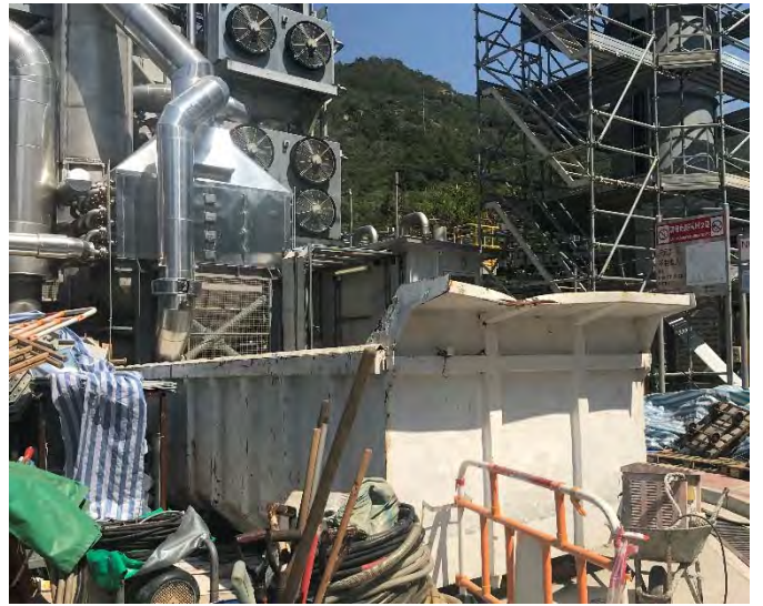
Construction waste skip was relocated.
