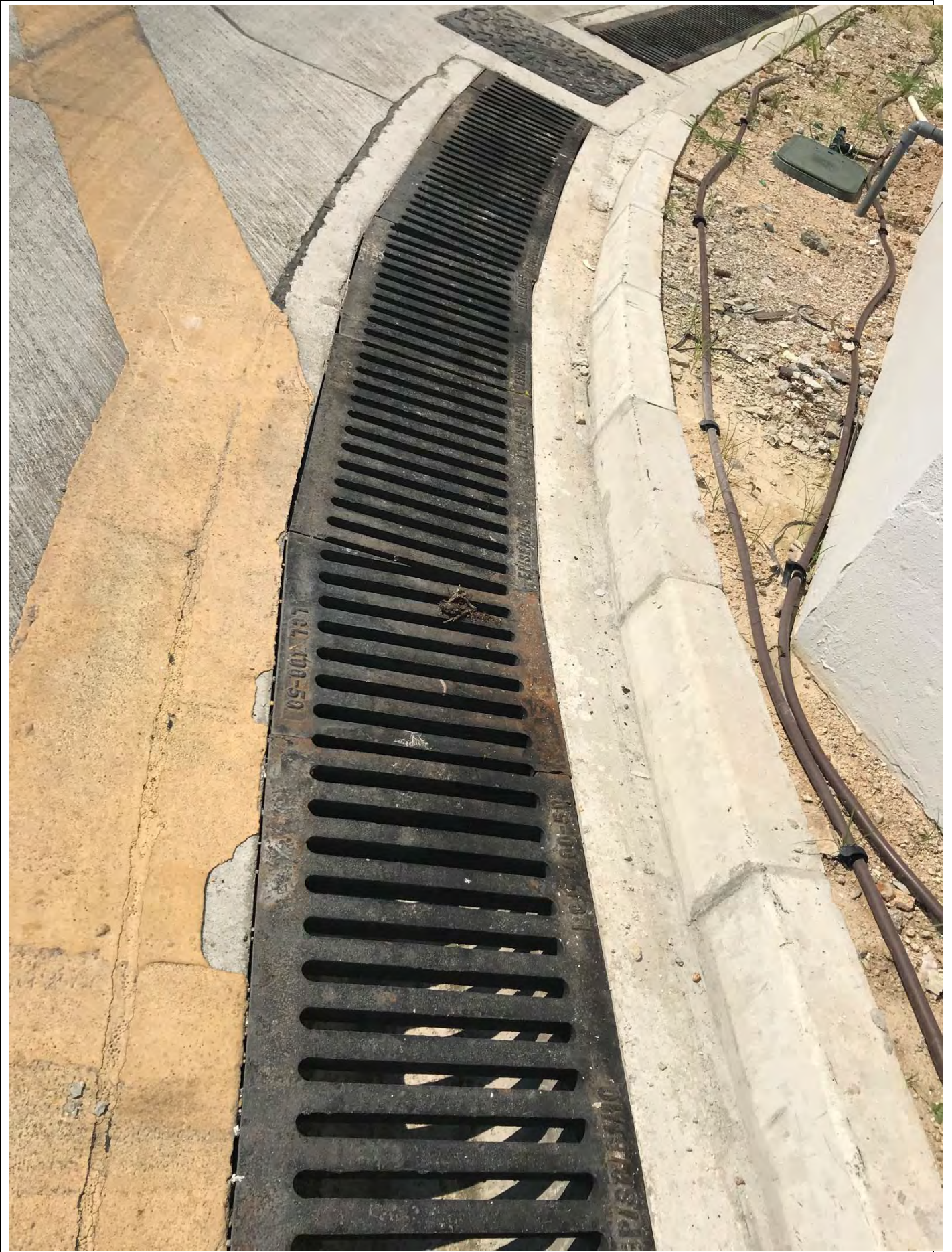
All surface channel
